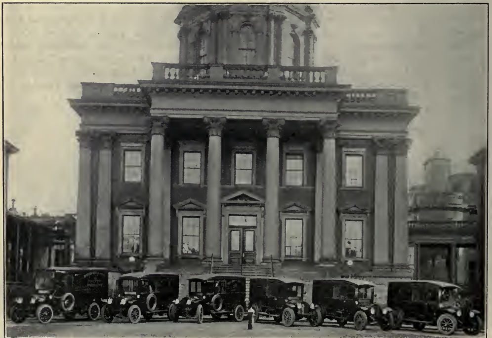
A GROUP OF AMBULANCES MADE BY THE WHITE COMPANY FOR THE SERVICE OF THE BOSTON CITY HOSPITAL
